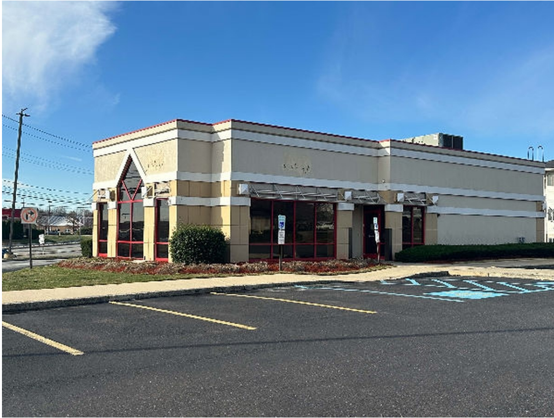
Building exterior and Egypt Road frontage — 2610 Egypt Road, Audubon, PA
